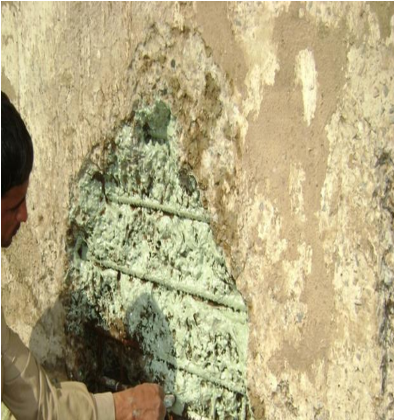
Applying Epoxy bonding agent
