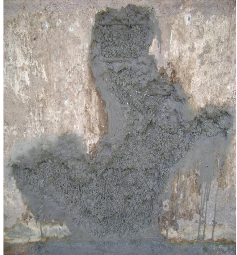
Concrete Repair with Mortar
