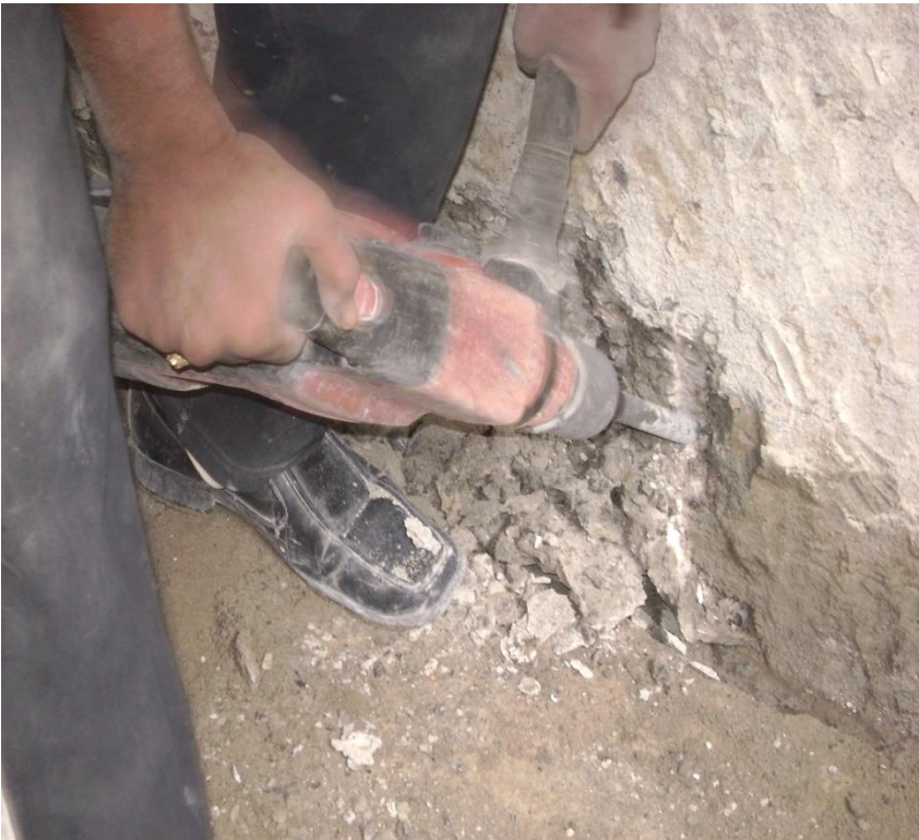
Step 1 (Chisel The Point)
